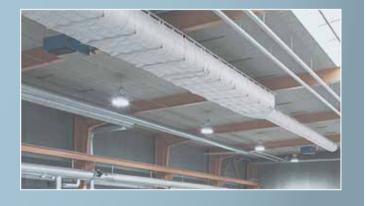
Rectangular ducts are typically created using internal membranes for structural integrity, and support hoops may be used on all four sides. This ensures that the duct keeps its profile when the air is turned on, despite the natural pressure toward bulging.
