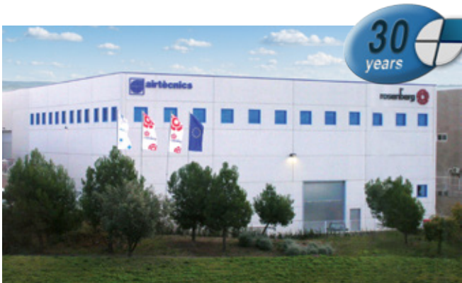
Airtècnics headquarters in Castellar del Vallès (Spain)
