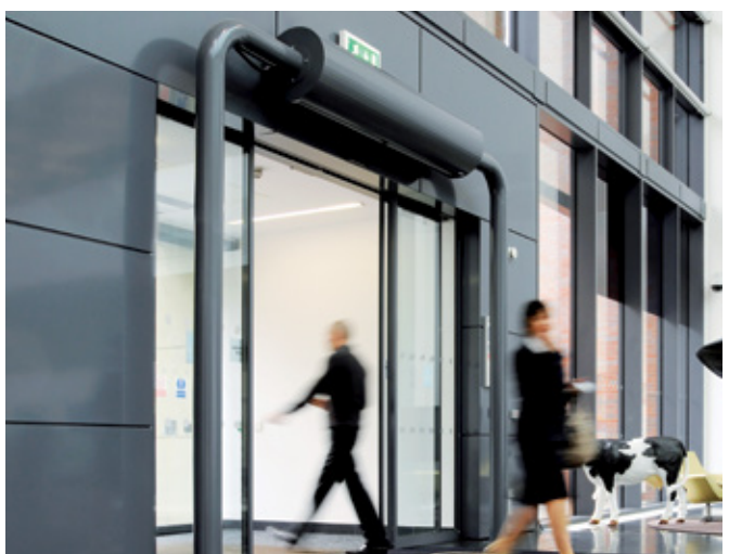
Rund Installation with special goalposts supports
