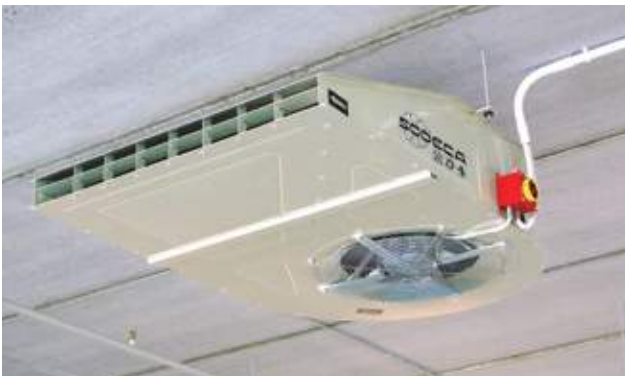
CI installed in car park
