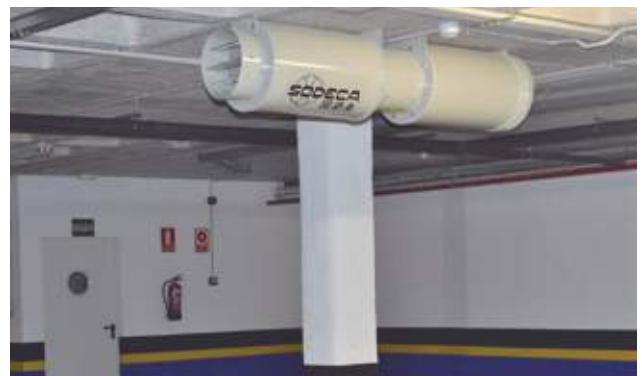
THT/IMP installed in car park
