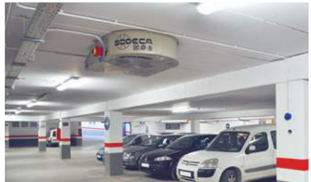
CI installed in car park
