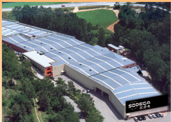
Headquarters of SODECA S.L.U., in Sant Quirze de Besora
